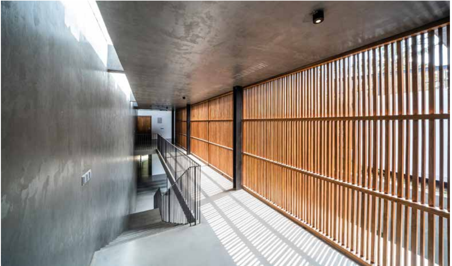
Timber screens and the random use of structural steel pillars along with cantilevered balconies create a sense of lightness to the concrete and masonry structure of the house
