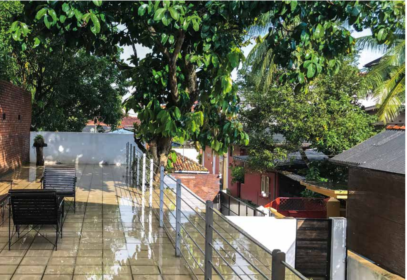
The uniqueness of the design extends as the existing Rose apple tree ( Syzygium jambos Alston) rooted at the entrance of the carport melds into the design through the open-air terrace slab, creating a free yet cosy atmosphere
